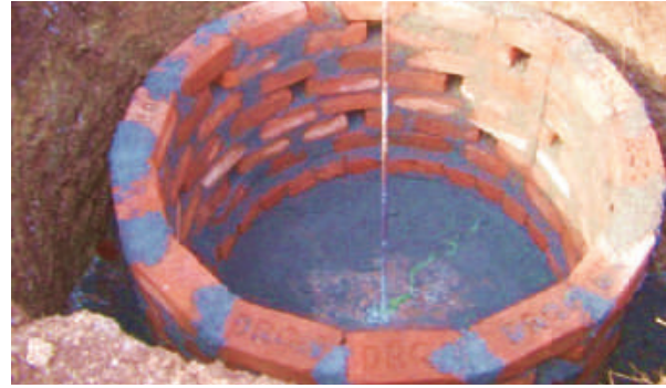
Upper layers in single brick with honeycombing in alternate layers
