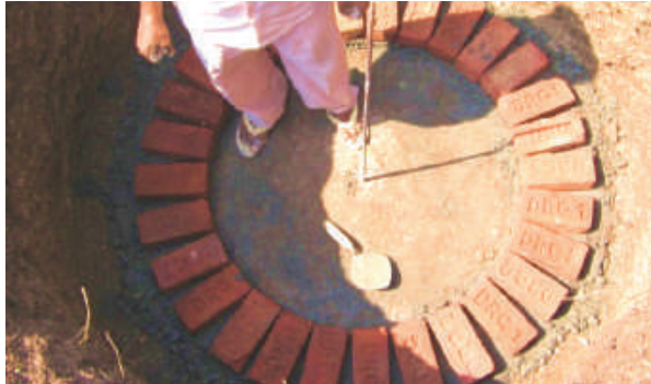
The first layer in 9" Brickwork
